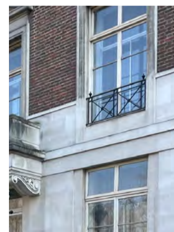
LIME STONE - re-used as flooring
