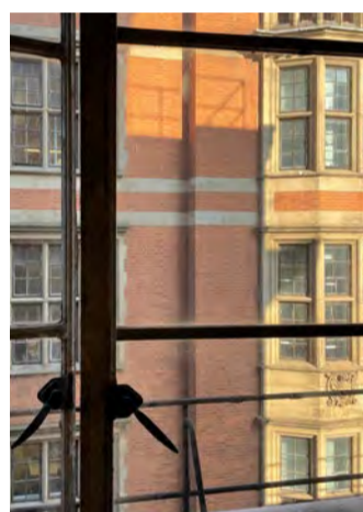
WINDOWS - re-used as interior walls
