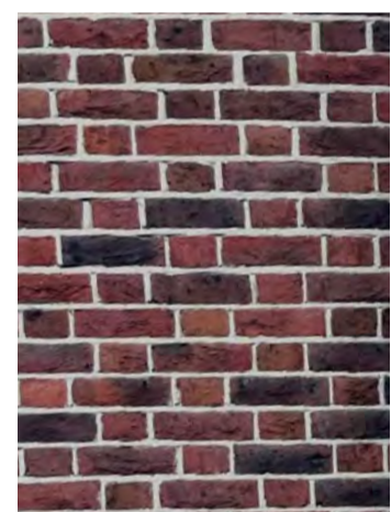
BRICK WALL - re-used in the facade
