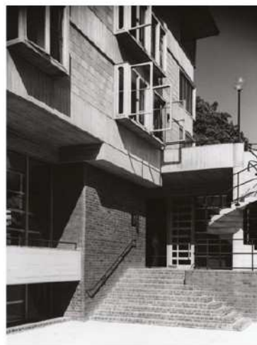
Cumberbatch Building (1966), Trinity College Oxford, by Macquire and Murray
