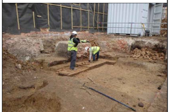
Wall 1016, looking south east
