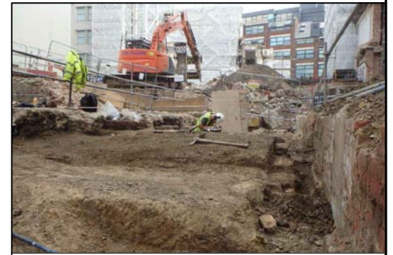
Layer 1581, looking north east
