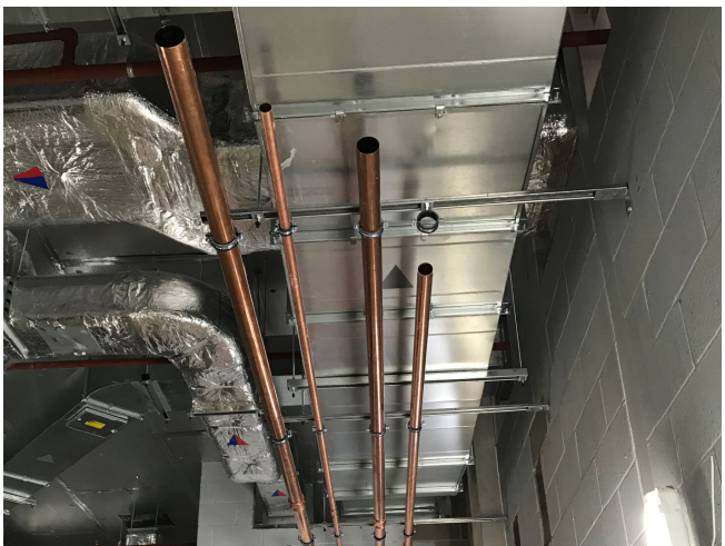
4. Modular mechanical services installation
