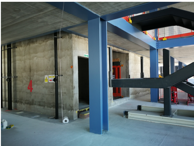
3. Internal exposed steelwork to Tower Building and academic stair
