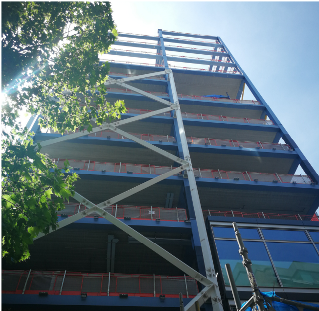
2. Super-structure works including the exoskeletal bracing and the cladding on the north elevation
