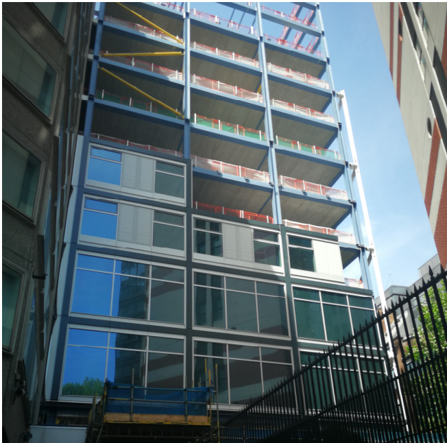
1. Cladding installation progress to the east elevation
