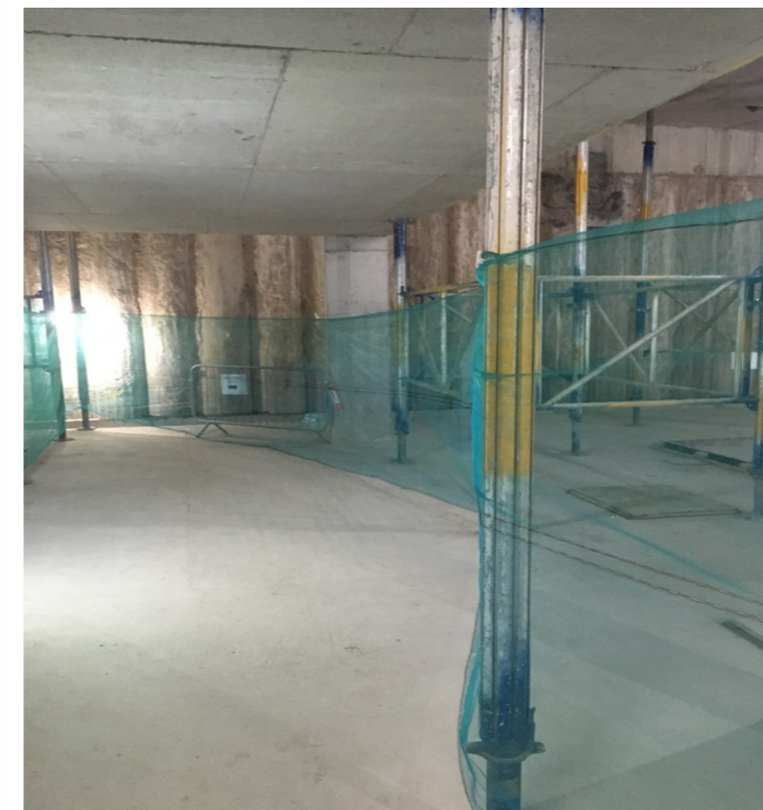
4. Basement level 1 works progressing
