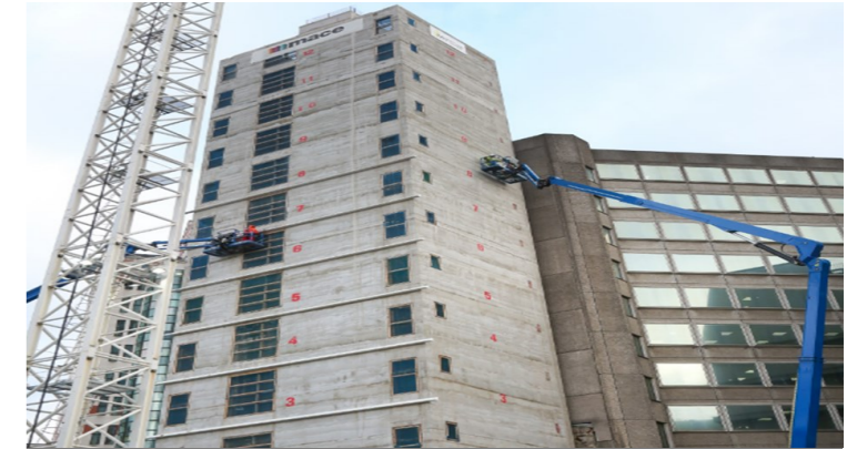
2. Billingtons install of angles.
