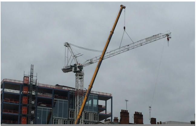
5. Tower Crane 1 removal – Main jib removal with a mobile crane.
