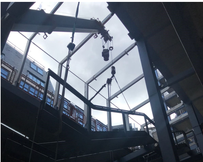
4. Atrium staircase steel work installation
