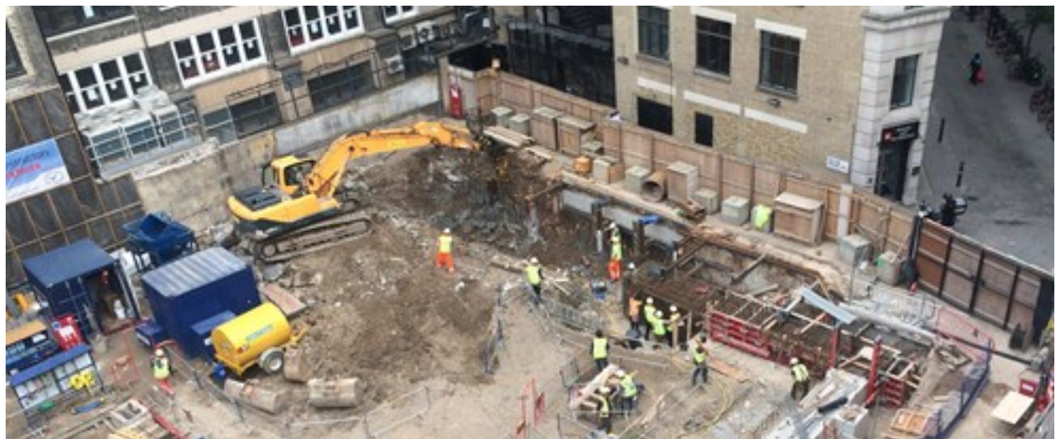
New Inn Passage capping beam
