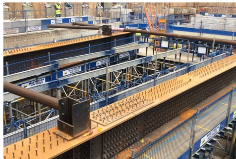
Falsework to plate girder beam
