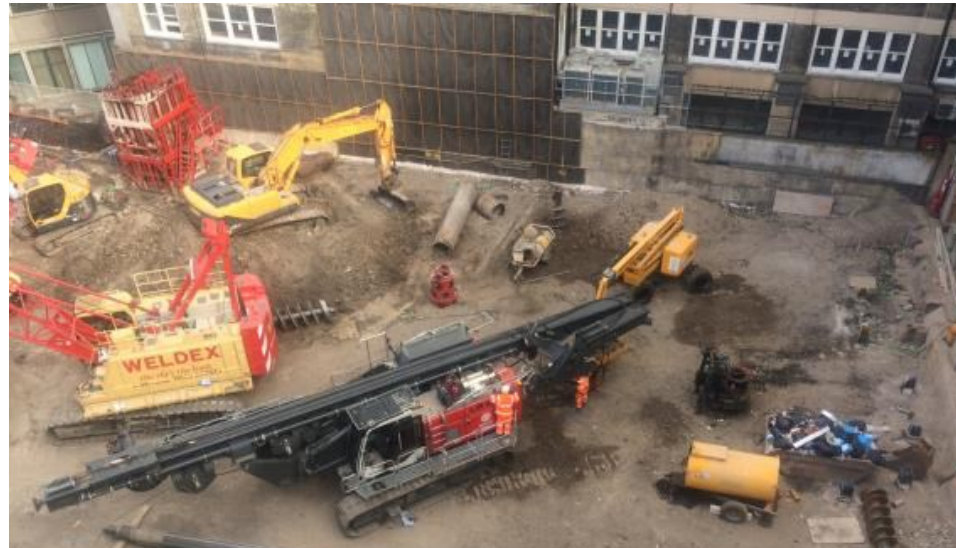
The LDA piling rig being dismantled
