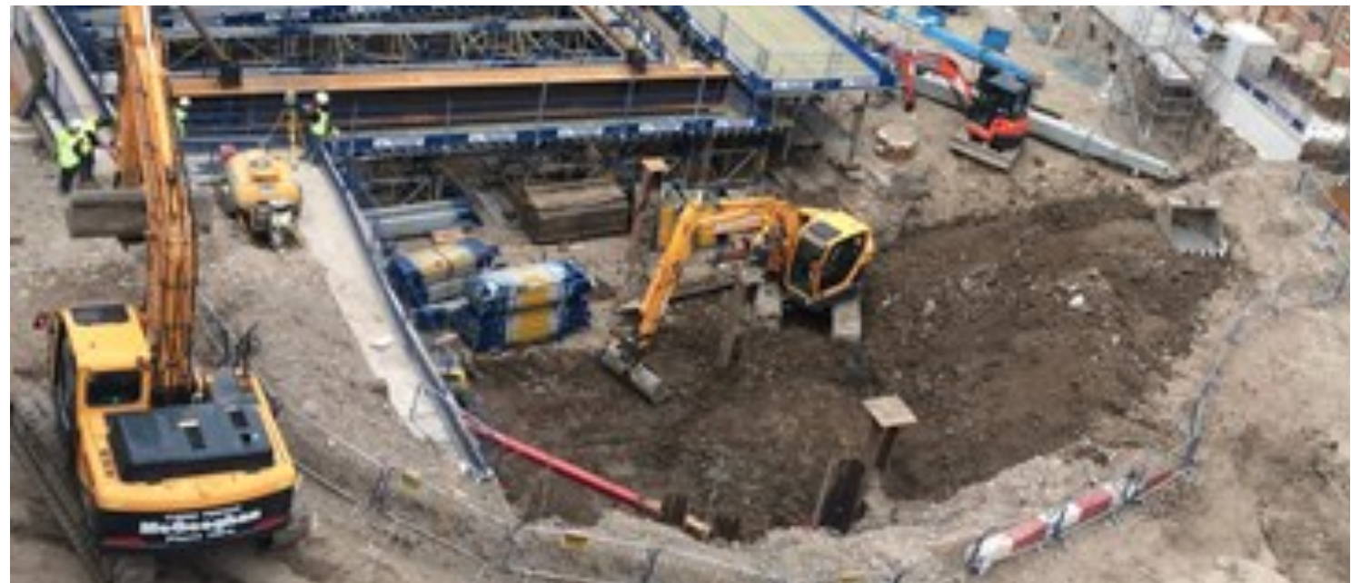
Top down construction - zone 1
