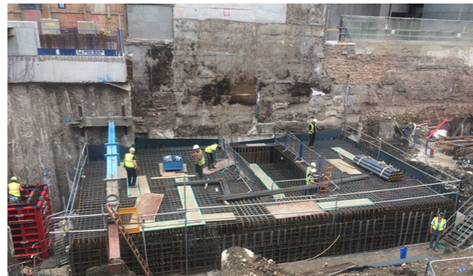
3. East core walls progressing at Basement level
