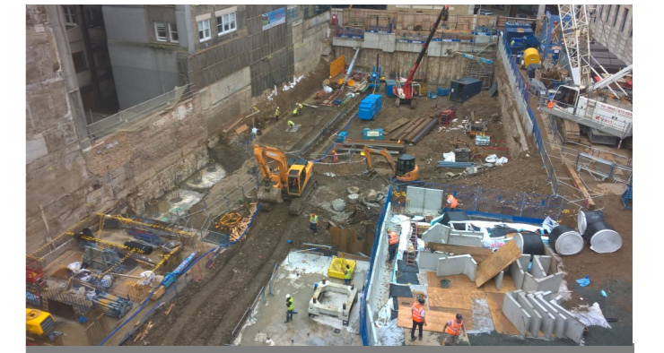
4. Site view from Mace phase 2 welfare set up
