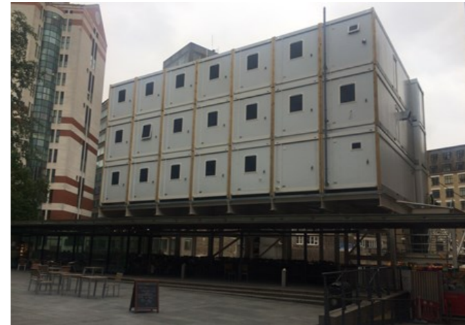
1. New Mace site offices
