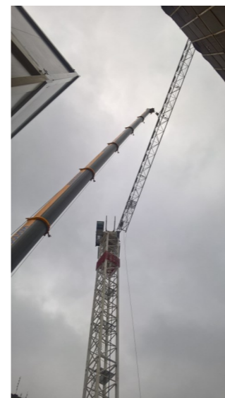
5. Tower Crane 1 (TC1) was installed on site.
