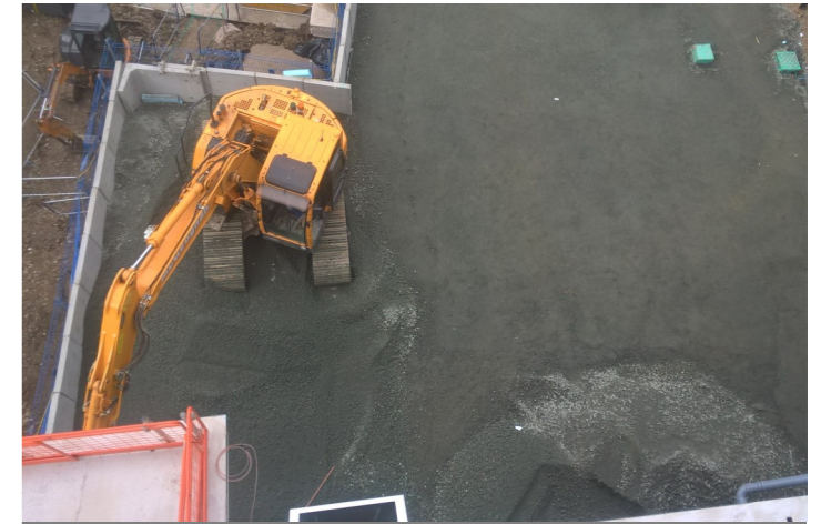
2. Top down slab being prepared for tarmac (now complete)
