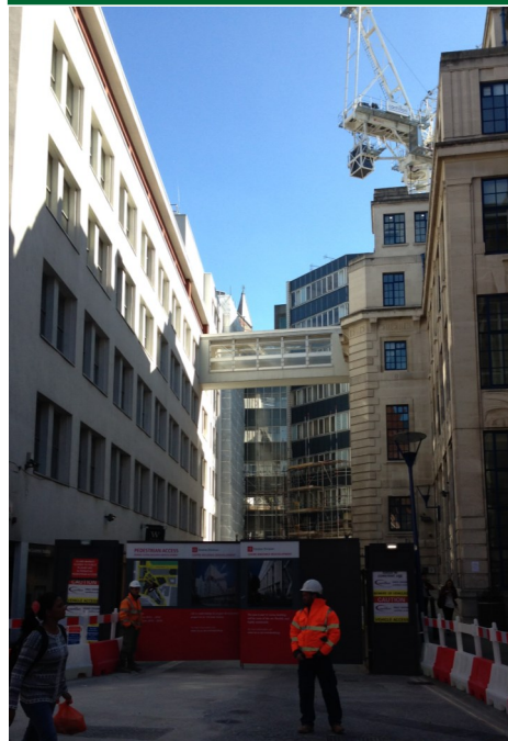
View of tower crane from Portugal Street
