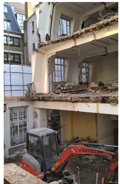
Clare Market demolition in progress
