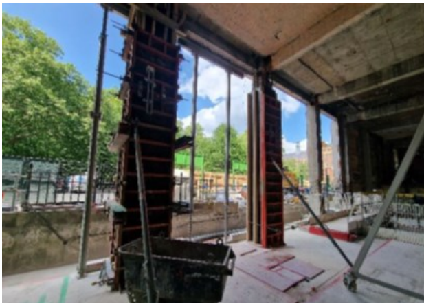
Ground floor column formwork
