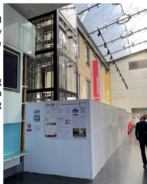
Hoarding Segregating Works from SSC
