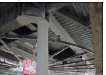
Agora primary steelwork
