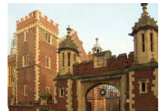
Gateway to Lincoln's Inn Library and Hall
