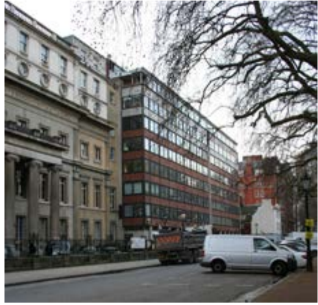
View of existing 44 LIF from Lincoln's Inn Fields
