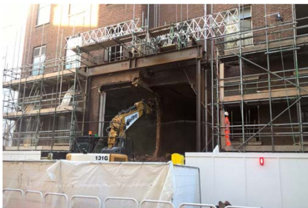
Fig 02 - Demolition Opening on Portugal Street
