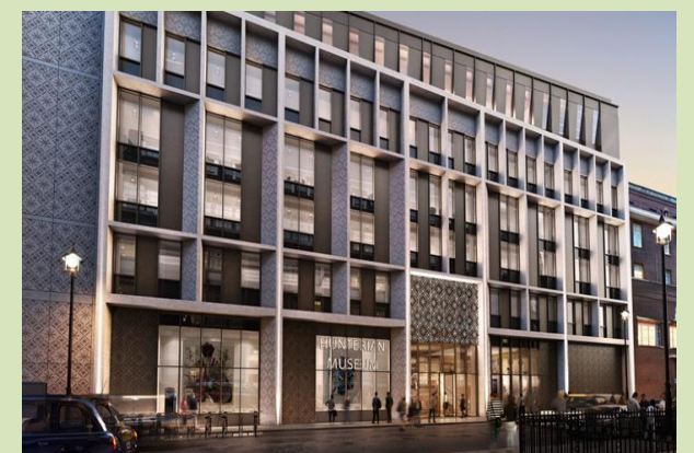
The planned new Portugal Street façade
