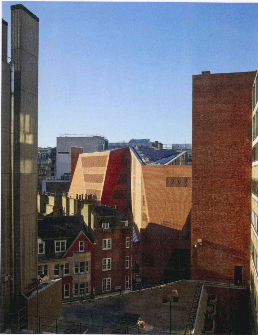
Left, below Hundreds of drawings were made for the hundred or so special bricks alone, which were hand-made by Coleford Brick & Tile and hand-laid by Swift Brickwork Contractors to precise assembly drawings made by the architects. The bricks are of a type usually specified for paving, chosen for its water resistance.
