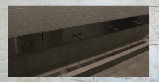
This footwash facility is fitted with auto sensor taps to activate water flow.
